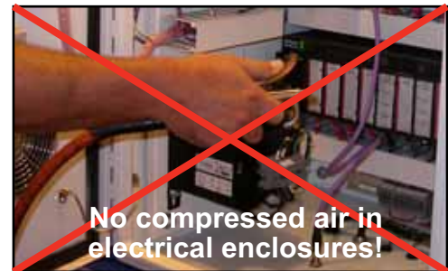
Figure 7-3: Never Use Compressed Air Inside an Electrical Enclosure
