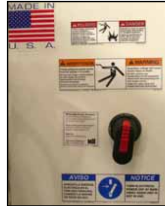
Figure 6-3: Disconnect Switch
